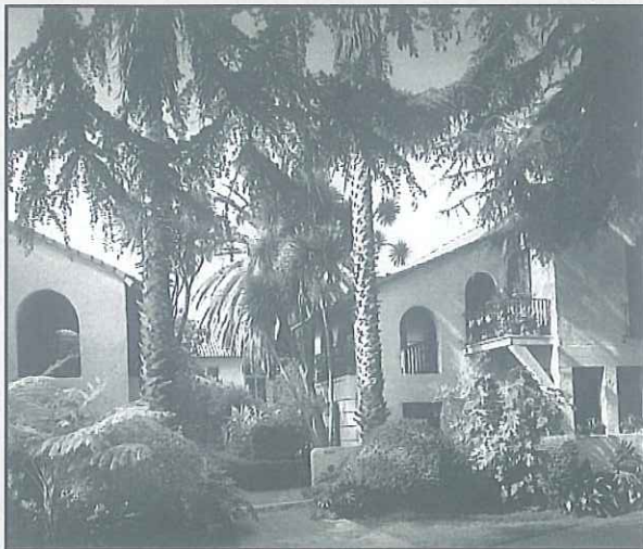
(below) Monterey Apartments in Los Angeles and (above) its open U-shaped plan (from Polyzoides et al., pp. 130-131)
