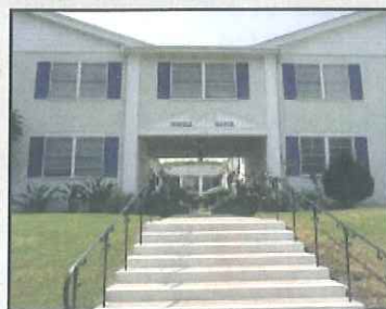
No. 415: Courtyard accessible from public right-of-way
